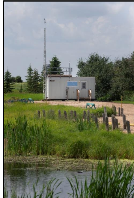
Figure 10: Range Road 220 Station
