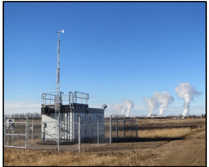
Figure 13: Scotford South Station
