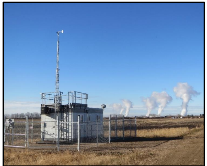
Figure 12: Scotford South Station
