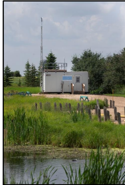
Figure 9: Range Road 220 Station
