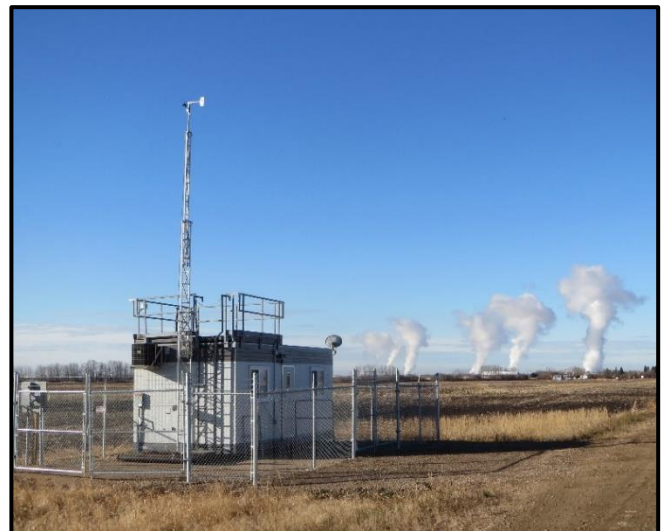
Figure 12: Scotford South Station
