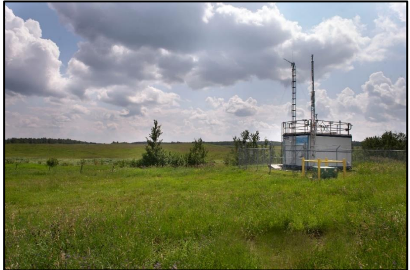
Figure 7: Lamont County Station
