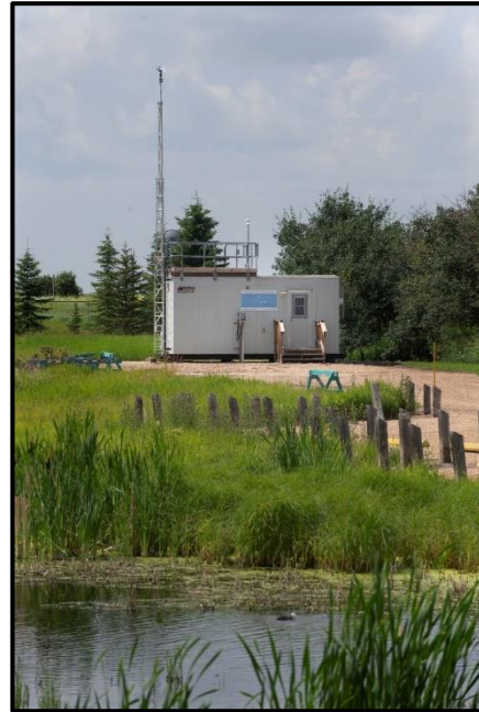
Figure 9: Range Road 220 Station
