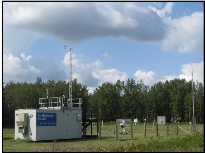
Figure 4: Elk Island Station
