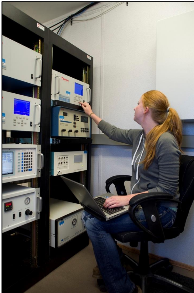
Figure 1: Continuous air monitoring station interior
