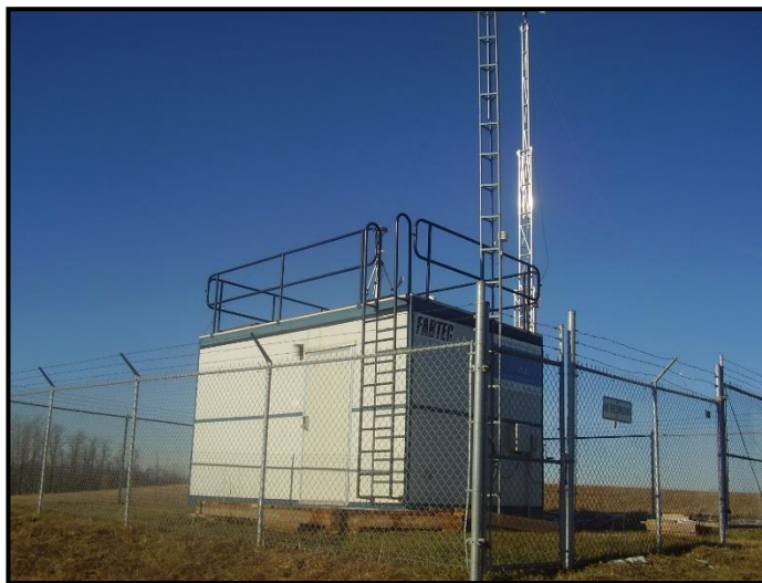
Figure 7: Lamont County Station
