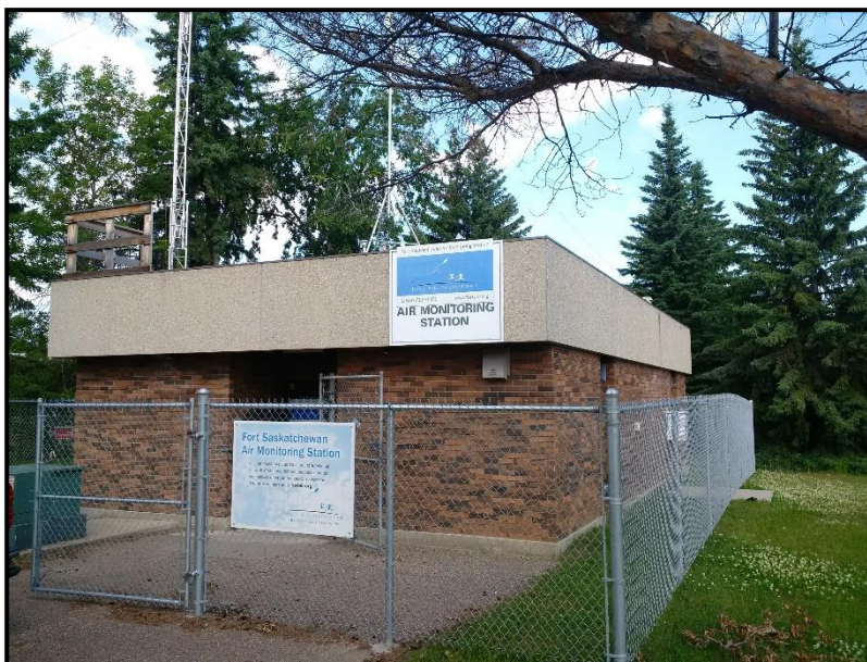
Figure 5: Fort Saskatchewan Station
