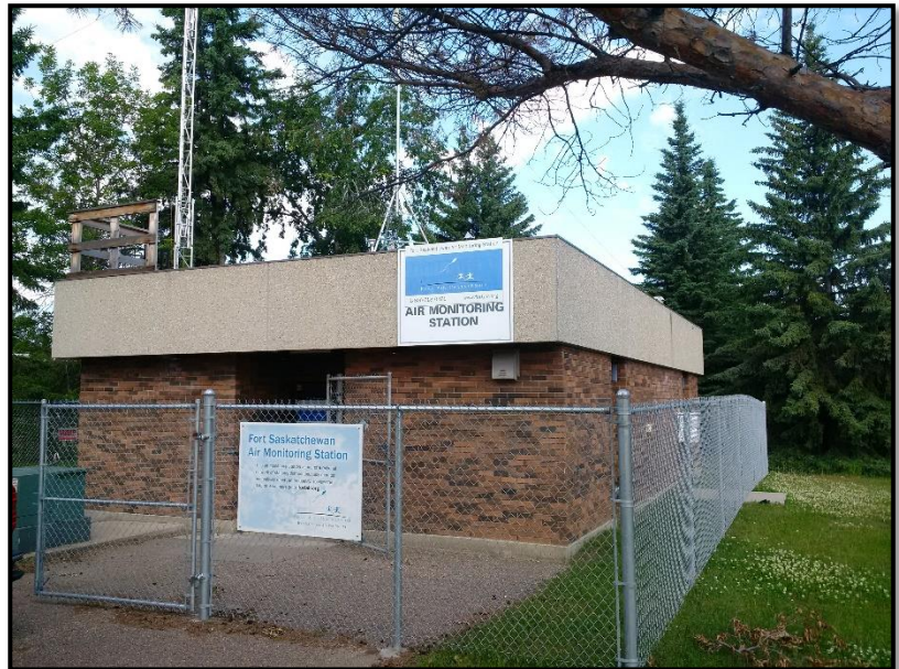
Figure 5: Fort Saskatchewan Station
